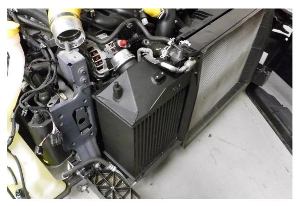
**21**. On some vehicles we have found the air conditioning pipe work can vary. If you find the air condition pipe is touching the back of the Forge intercooler very slowly and carefully bend the alloy pipe away from the intercooler.
