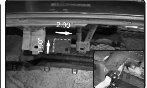
12. Locate the plastic panel inside the bumper, in between the two upper brackets. Measure 1.50" in and 2.00" right and draw cutting marks similar to the photo illustration. Use a suitable cutting device and cut on the marked lines.
